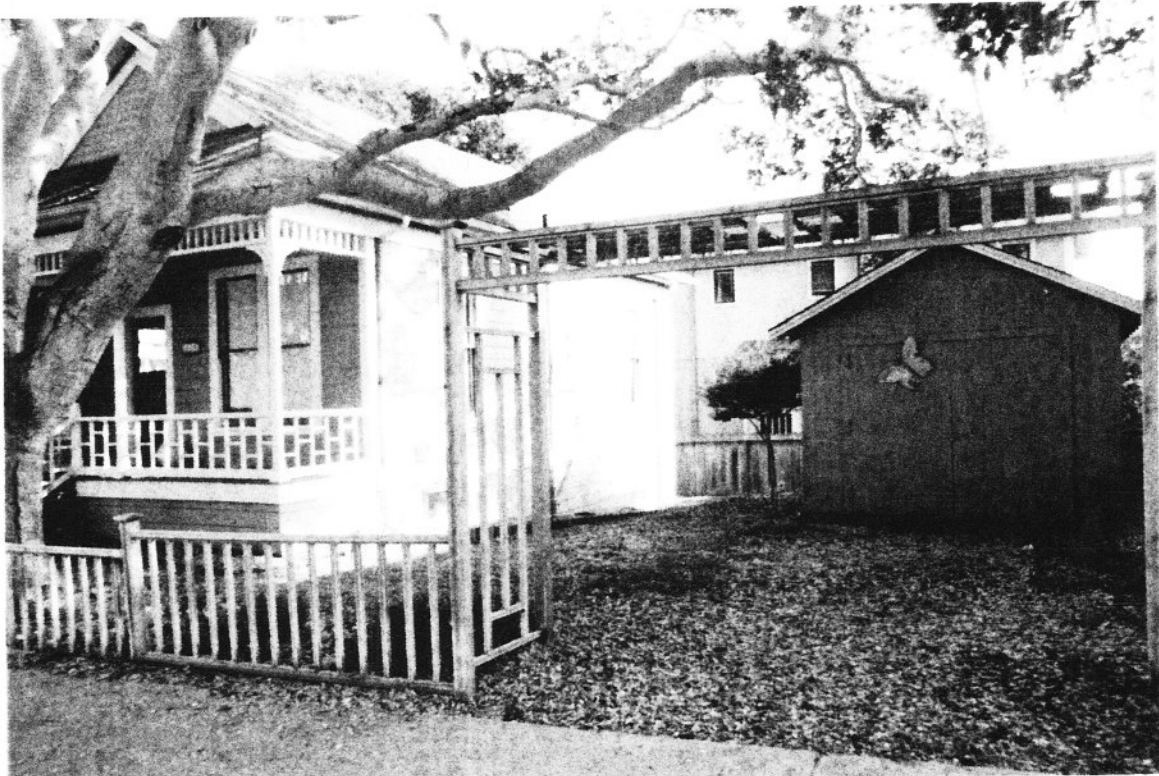
Photo #3. Looking NW at the south side-elevation, December, 2013.
