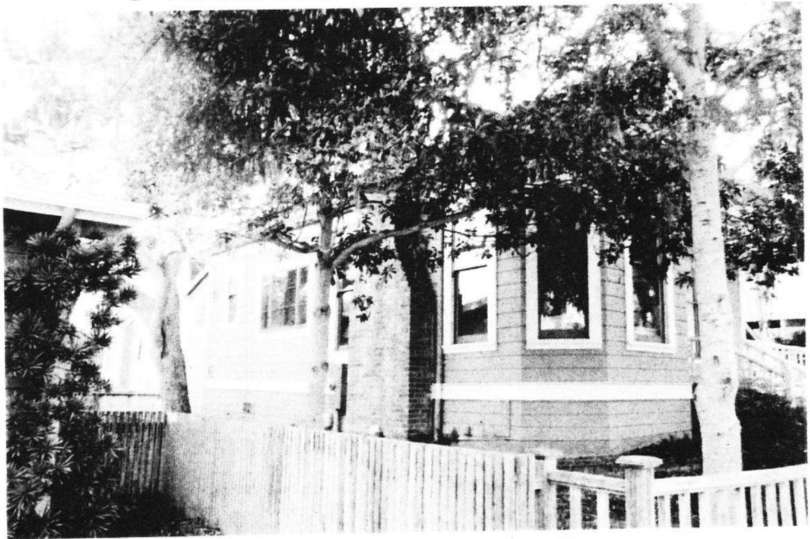
Photo #2. Looking SE at the north side-elevation. Note the more modern window, Dec., 2013.
